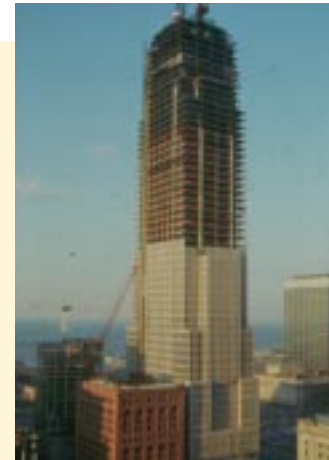
When construction of speculative office buildings slowed in the early 1990s, use of high-strength silica fume mixes dwindled as well.
